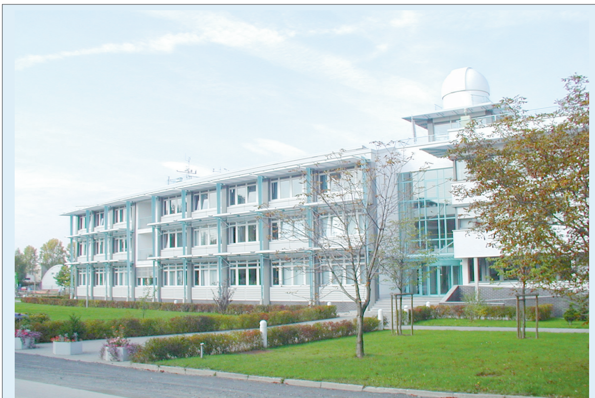
Fig. 1: IfT main building.
